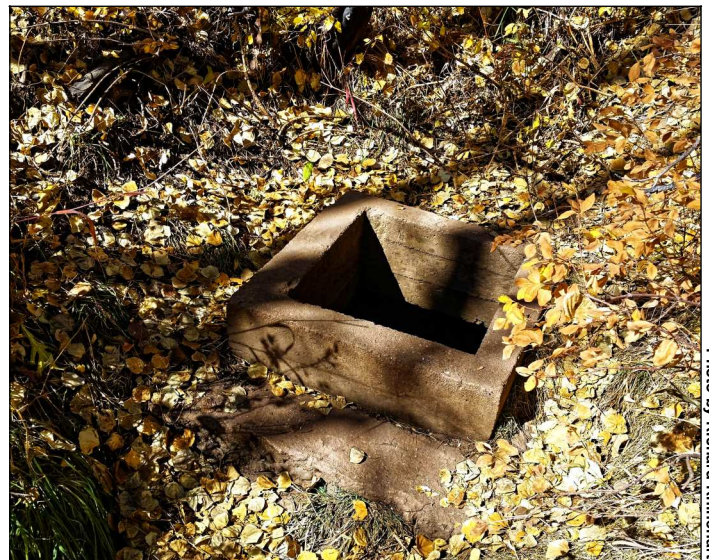
Old concrete work at the Transfer Spring.
